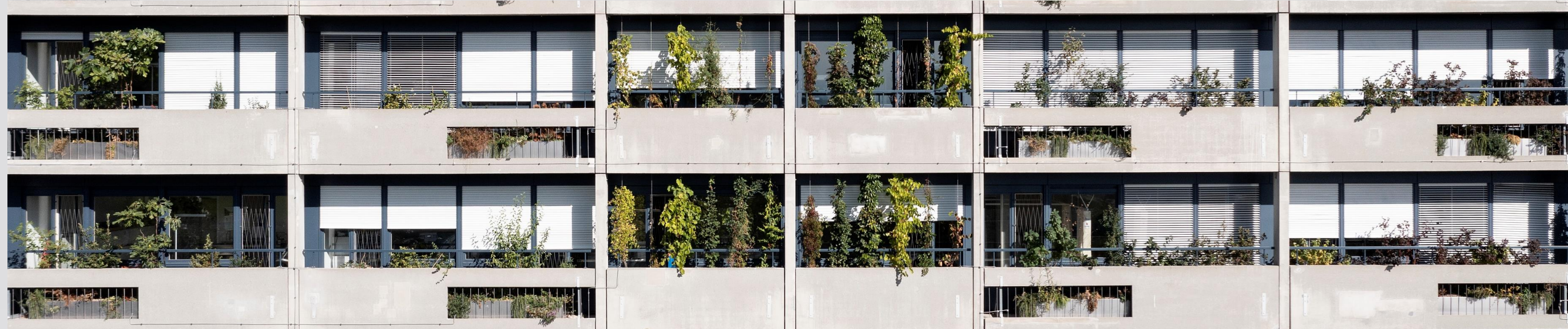
Figure 1. Green façade on the South side of the Triemli Hospital. Photo: Gaëtan Bally
