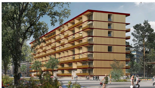
Fig. 1. Illustration of the reference building (source: UNAS Technology SA).
