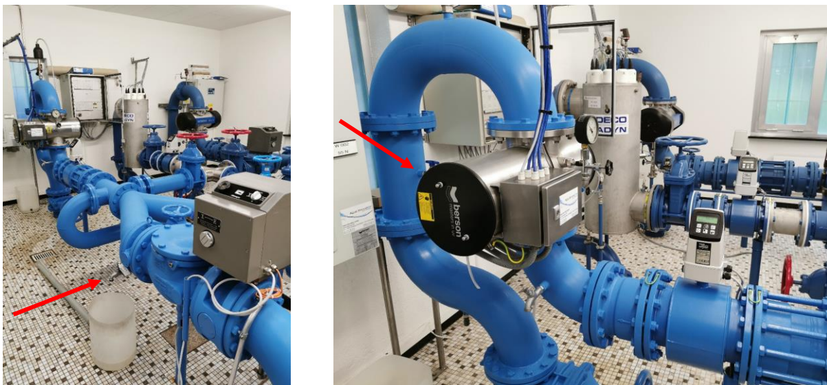
Figure 17: From left to right; Groundwater sampling site, marked with a red arrow, in Bischofszell; Sampling after UV-disinfection, marked with a red arrow. (Source Erb Severin)
