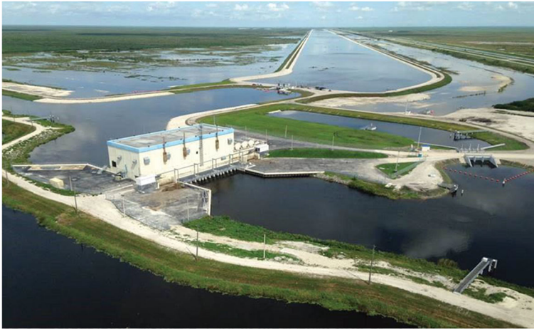
Fig. 3 A flow equalisation basin (FEB) designed to temporarily capture and hold stormwater runoff for release to the Florida Everglades stormwater treatment areas (STAs). By tempering flow rate, FEBs help maintain desired water levels in the STA and assist in optimising performance of stormwater treatment areas in removing phosphorus [59]
