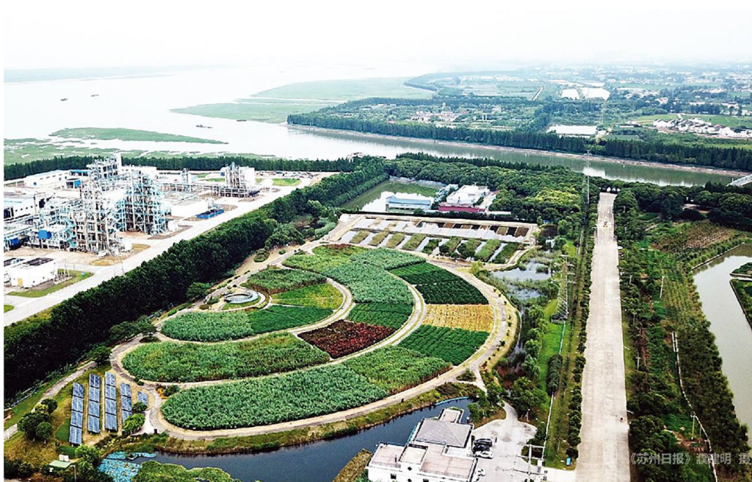
Fig. 6 Layout and performance of the industrial wastewater treatment constructed wetland
