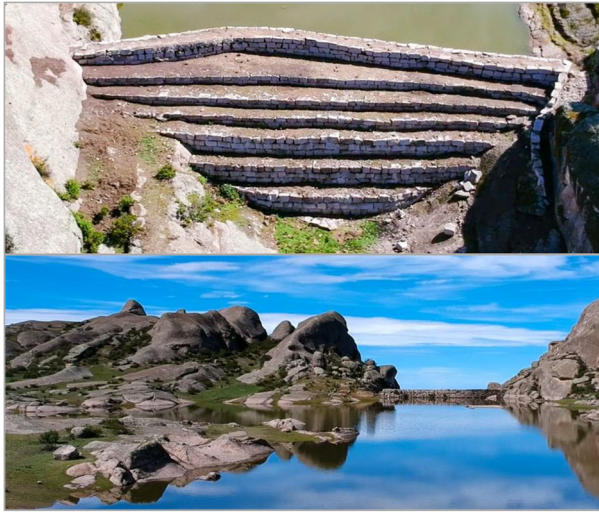
Fig. 5 Dike built of the Cachu-Cachu lake artisan reservoir: At the top of the front view and at the bottom of the rear view of the dike and the Cachu-Cachu pond
