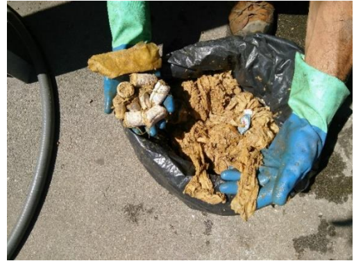
Figure 22 Wet wipes and tampons fished out first chamber of septic tank Source: Pravin G. Moorthy
