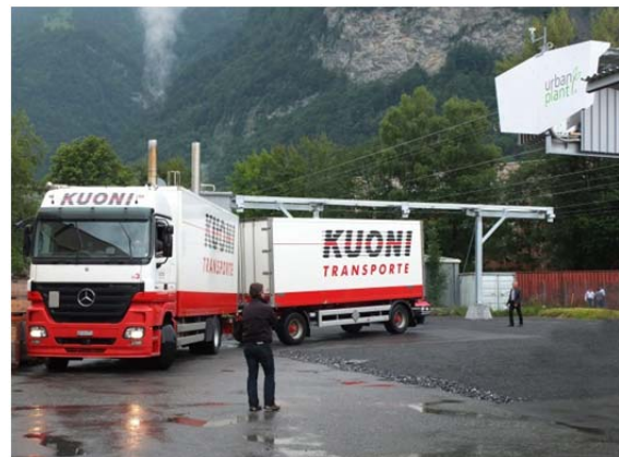
Figure 8: Urban Plant UP 50 in Balzers (Top power and shade; bottom a truck is passing below the PV plant).
